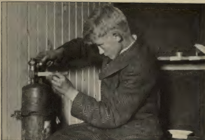
FIG. 46. The expansion of the compressed gas freezes the moisture on the tube.
